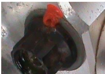
Figure 13 - Torque seal installed
